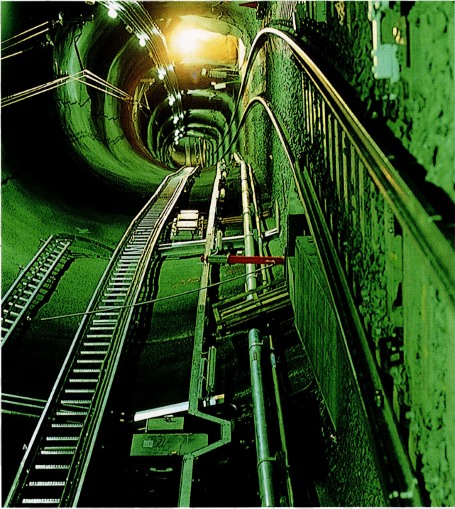
Driven tunnel on approach to the station.
